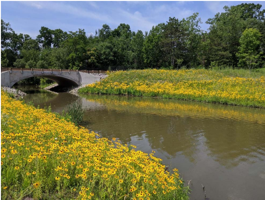
Completed open connection between the Rouge River and the Oxbow wetlands, with the natives in bloom.
