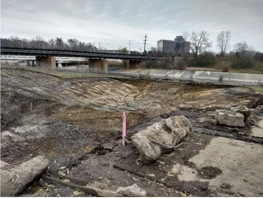
Initial construction of the open cut connection between the Oxbow wetlands and the Rouge River.
